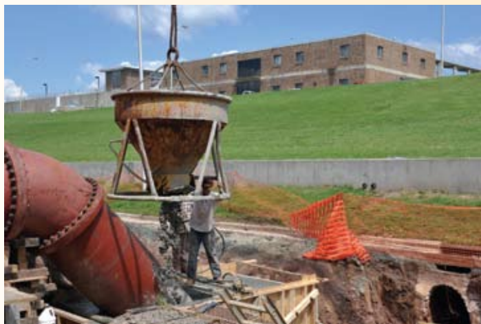
Installation of the New Brown WTP 42 inch Distribution Line
