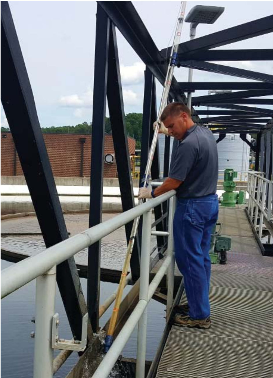
North Durham Water Reclamation Facility Superintendent John Dodson collects a sample from a secondary clarification tank.
