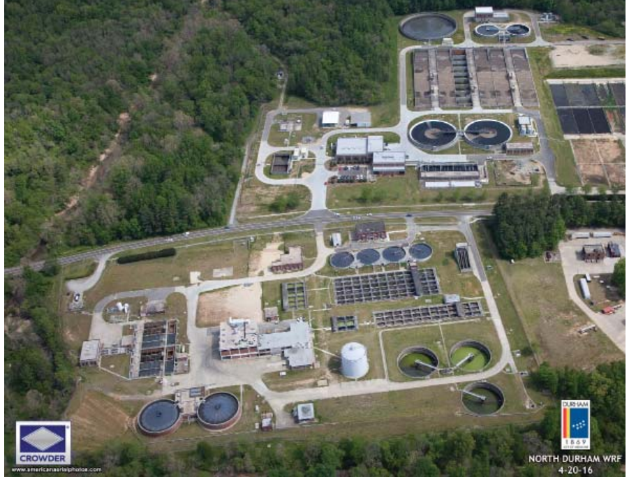
North Durham Water Reclamation Facility. The City operates two WRFs.
