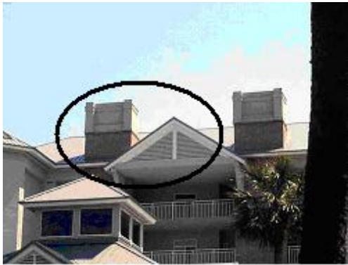
Concealed Equipment units – Concealed Antenna
