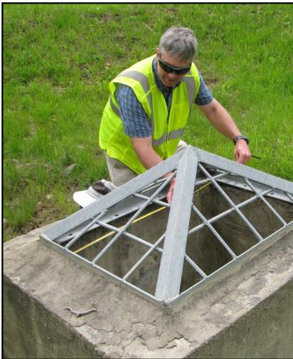
*Engineering Technician Bill Hailey measures part of a stormwater control device in Little Lick Creek watershed.*
