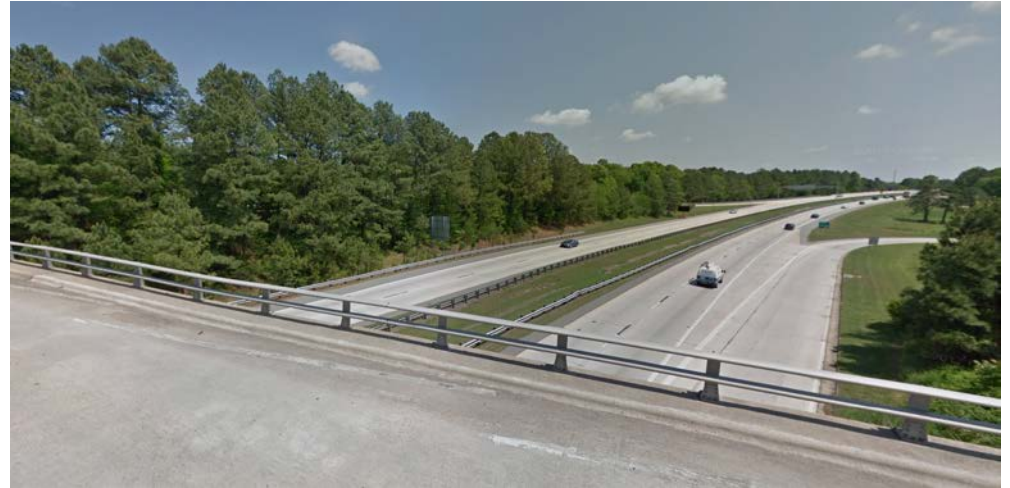
Looking east at the Durham Freeway from Briggs Ave overpass
