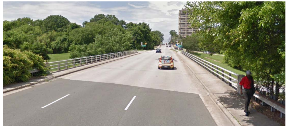
Looking north at Duke St overpass
